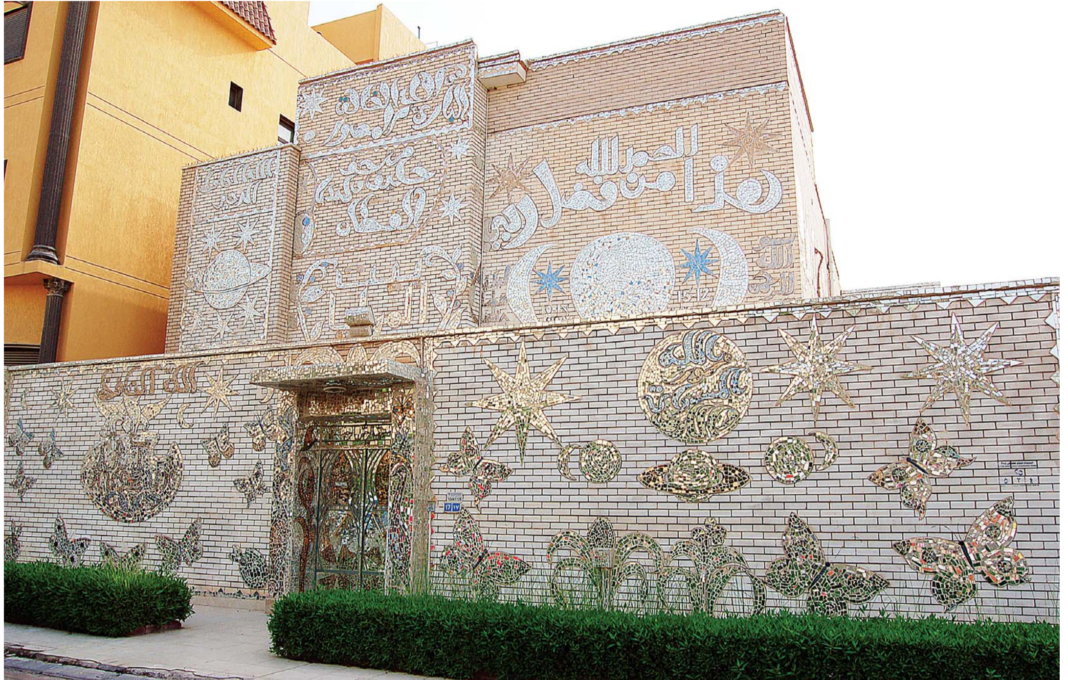
KUWAIT: The House of late artist Khalifa Al-Qattan and Lydia Al-Qattan. The house is built without windows and inlaid with glass and ceramics. The house is an artistic masterpiece. —KUNA
