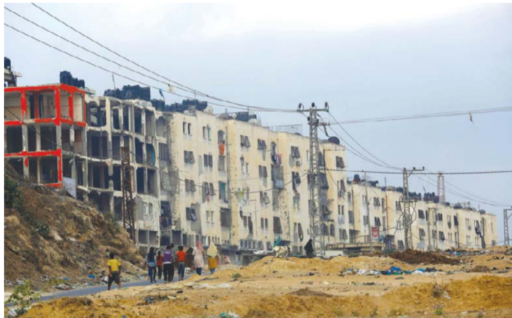
BEIT HANUN: Palestinians walk near buildings which were destroyed during the 50-day war between Israel and Hamas militants in the summer of 2014 in Beit Hanun. — AFP
