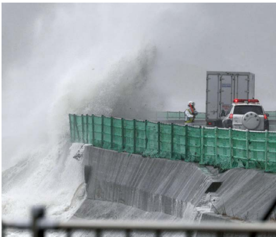
MIYAGI: Waves crash against a coastal road in Minamisanku, Miyagi prefecture, northeastern Japan yesterday. — AP
