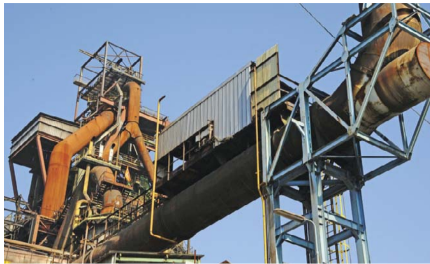
HAYANGE: Photo shows blast furnaces of steel giant ArcelorMittal at the Florange site, in Hayange, eastern France. — AFP
