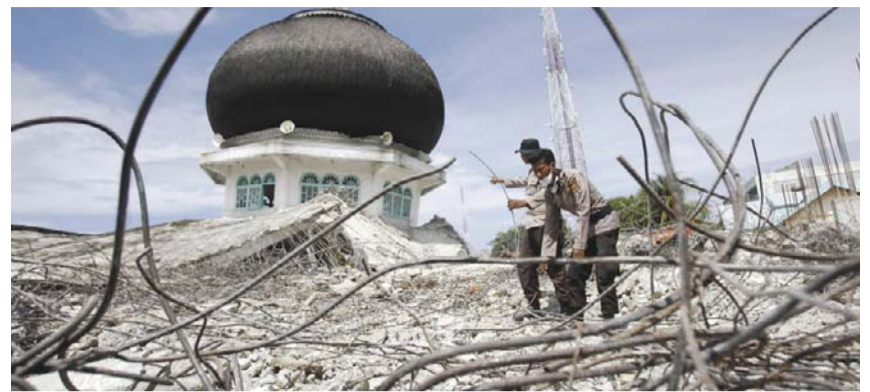
ACEH: Police officers help clear rubble at the ruin of a mosque collapsed in Wednesday's earthquake. — AP
