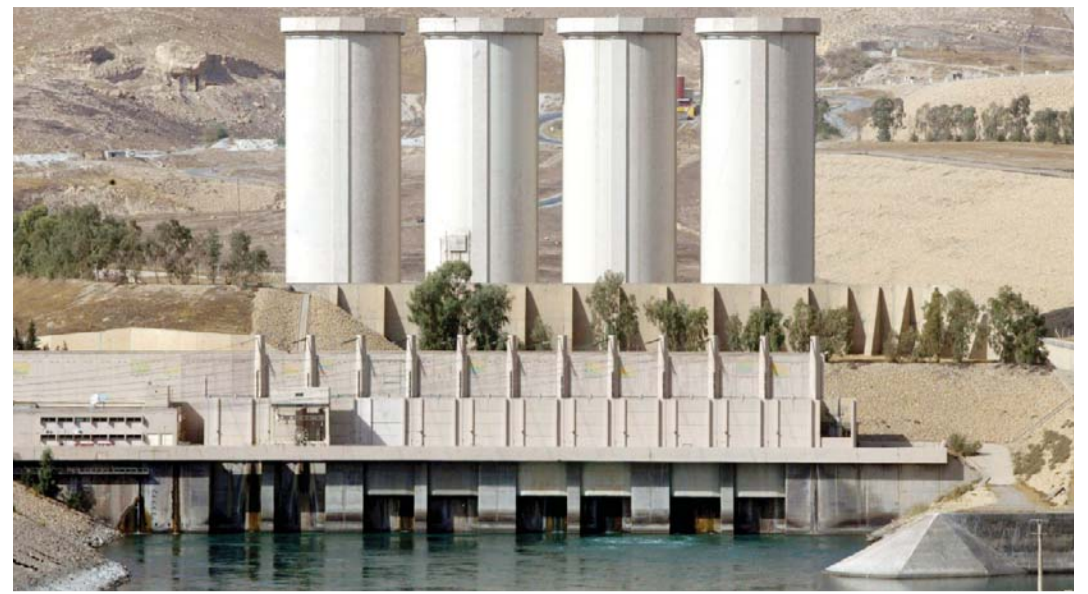
Photo shows a general view of the Mosul dam on the Tigris River around 50 kilometers north of the northern Iraqi city of Mosul. Iraq announced yesterday that it has awarded Italian firm Trevi a contract for the repair and maintenance of the country's largest dam, which is in danger of catastrophic collapse. — AFP
