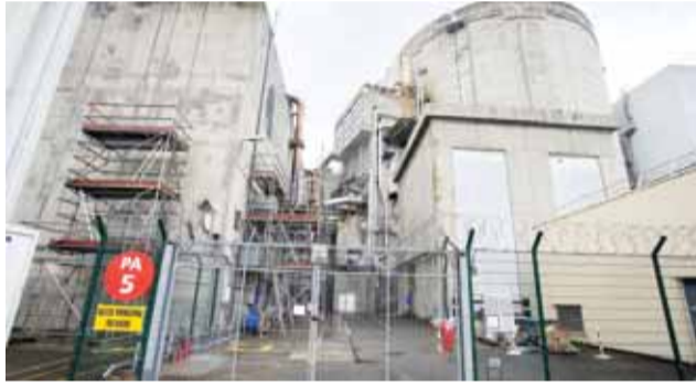
FESSENHEIM, France: This file photo taken on April 09, 2013 shows a reactor of the Fessenheim nuclear power plant. — AFP
