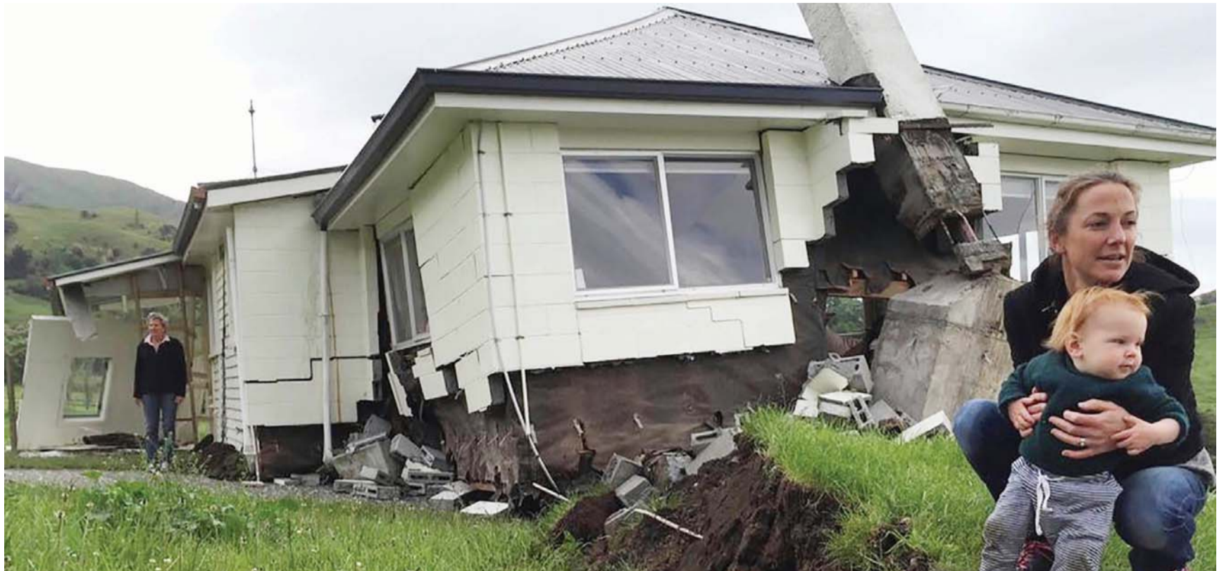
BLUFF STATION, New Zealand: A woman and child are seen in front of a house damaged by an earthquake as it sits on the fault line near Kaikoura on the South Islands east coast. —AFP
