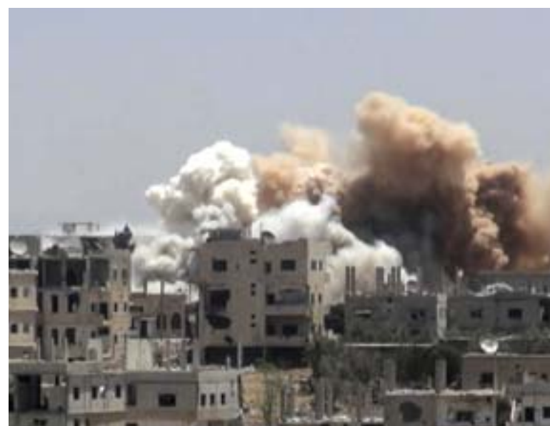
DARAA, Syria: This frame grab from video provided yesterday shows smoke rising over buildings that were hit by Syrian government forces bombardment. — AP
