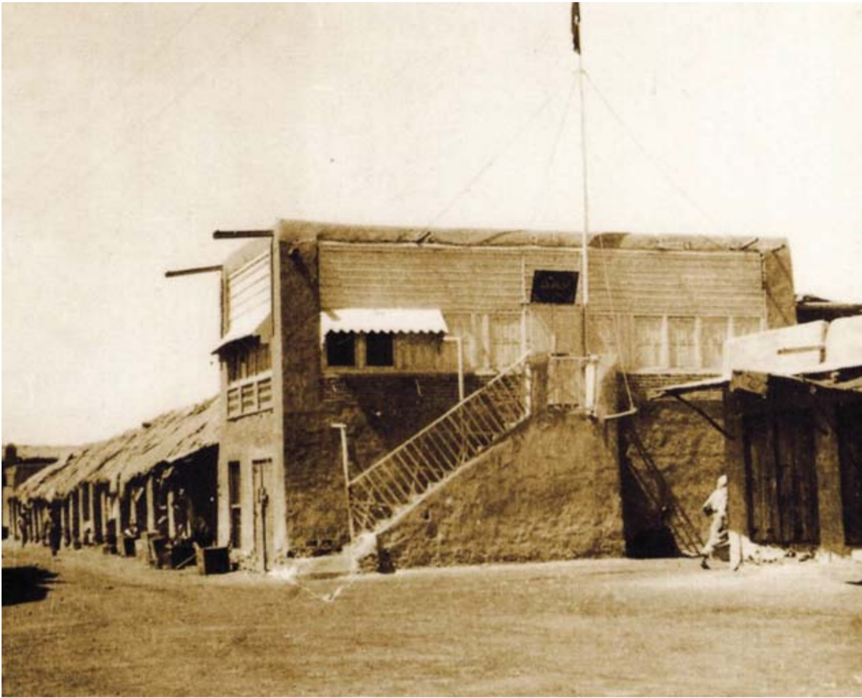
The Sheikh Mubarak Kiosk, one of the most important historical places in Kuwait. Founded in 1897 Kuwait's seventh ruler Sheikh Mubarak Al-Sabah(1840 -1915), it was regarded as the seat of government, where Sheikh Mubarak used to sit in the morning and monitor the affairs of government. The kiosk was surrounded by a variety of markets such as the vegetable, dates and water markets. The state renovated and officially reopened the kiosk as a tourist attraction in 2011. (Source: Sons of Sindbad, the Photographs, by Yacoub Hijji and Grace Pundyk, London, 2006. Prepared by Mahmoud Zakaria Abu Alella, heritage researcher in the Ministry of Information)
