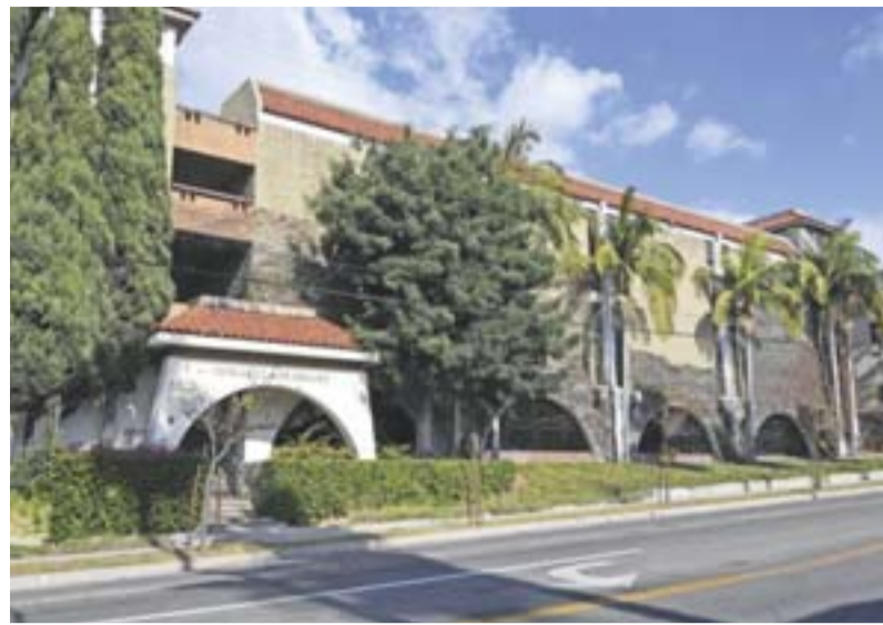
An exterior view of the Immaculate Heart High School in Hollywood, California where actress Meghan Markle was educated.
