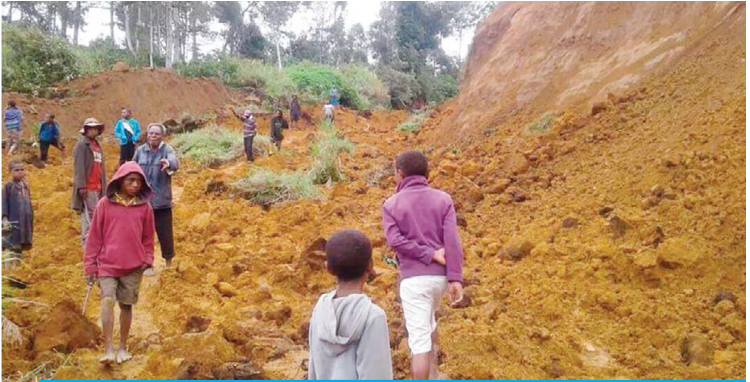
NIPA, Papua New Guinea: People walk at the site of a landslide near the village of Ekari in Papua New Guinea's highlands region after a 7.5-magnitude earthquake. — AFP
