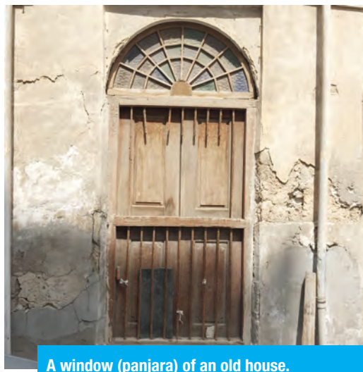
A window (panjara) of an old house.
