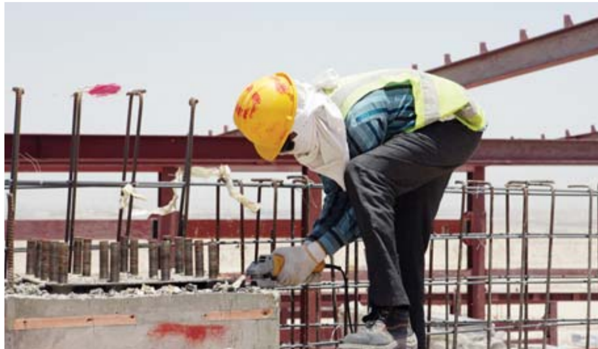
KUWAIT: This archive photo shows a laborer working at a project's site in Kuwait. This photo is used for illustration purpose only.
