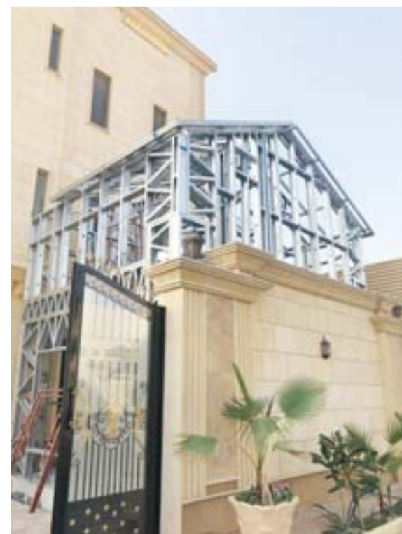
Galvanized steel is used to add a second floor at a house in Kuwait.
