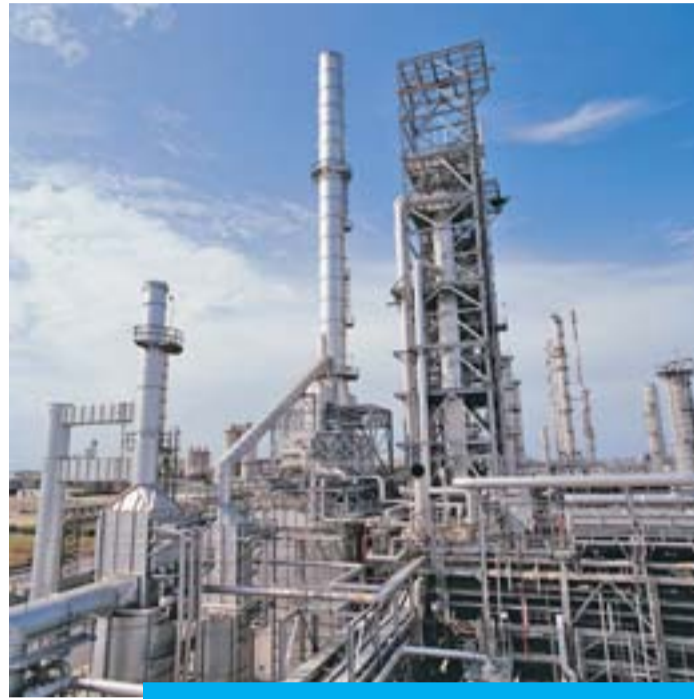
KUWAIT: Expansion works at Al-Zour refinery. — KUNA
