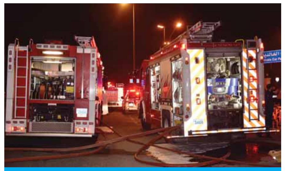
KUWAIT: A power transformer at Kuwait University's Khaldiya campus caught fire Sunday night. Industrial Shuwaikh and Shuhada fire station responded and put out the blaze. No injuries were reported. — By Hanan Al-Saadoun
