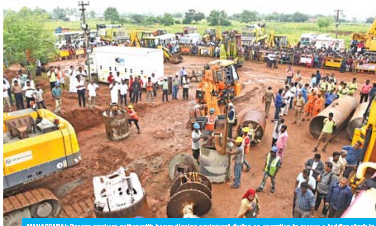
MANAPPARAL: Rescue workers gather with heavy digging equipment during an operation to rescue a toddler stuck in a deep well near Manapparal town in Tiruchirappalli district, in India's southern Tamil Nadu state yesterday. — AFP
