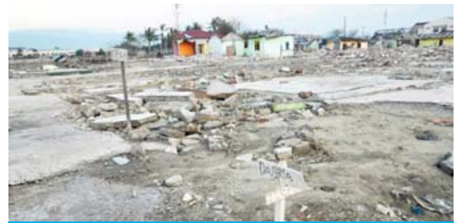
PALU, Indonesia: The remains of buildings are seen on a neighborhood area affected by liquefaction-a process where the ground starts behaving like a liquid due to the September 28, 2018 earthquake, in Palu. — AFP
