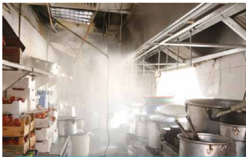
KUWAIT: The restaurant's kitchen after the fire.
