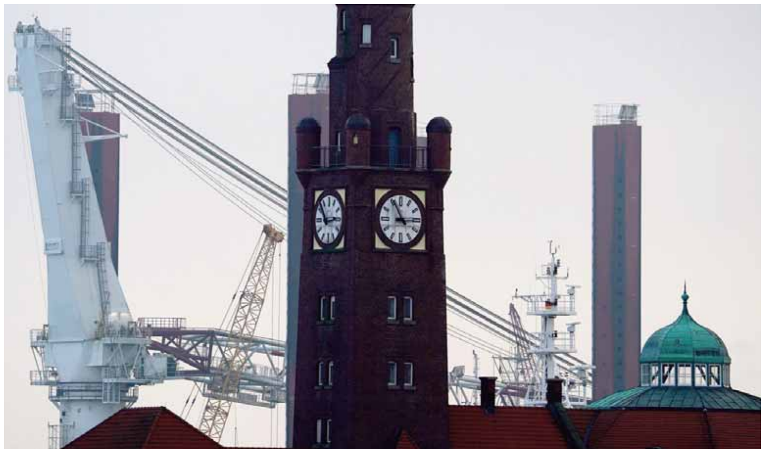
Cranes are seen at the quay at the harbor CuxPort at the North Sea in Cuxhaven, northern Germany. As most of the trade handled here is with the UK, Cuxhaven is perhaps the most sensitive port on the German side affected by post-Brexit-trade. — AFP
