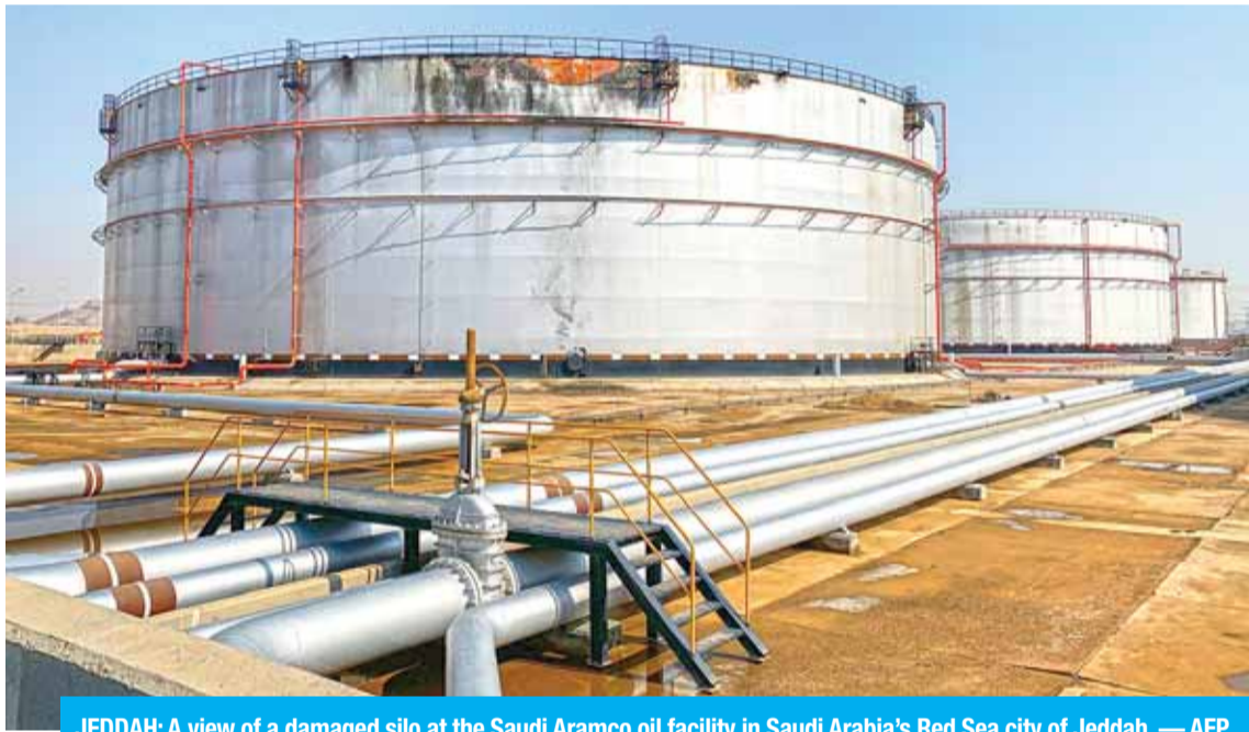
JEDDAH: A view of a damaged silo at the Saudi Aramco oil facility in Saudi Arabia's Red Sea city of Jeddah. — AFP
