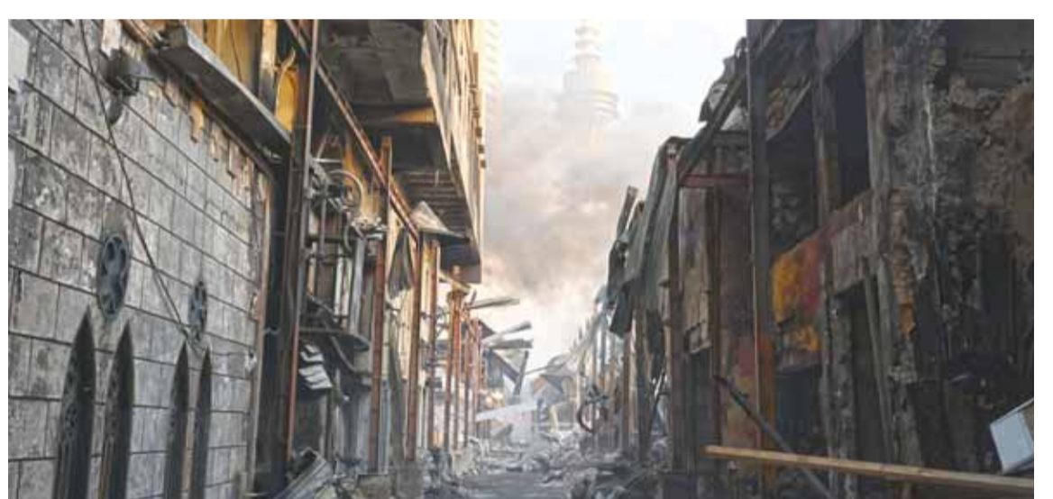
Heavy damage in Souq Mubarakia as the Liberation Tower is seen in the background.
