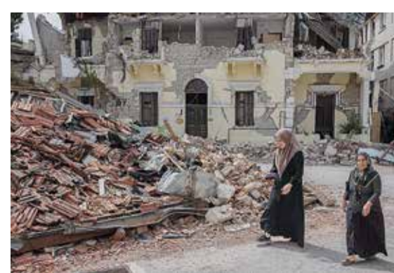
HATAY, Turkey: Women walk past the ruins of buildings on May 22, 2023 in one of the cities worst affected by the devastating earthquakes that hit southern Turkey earlier in the year. — AFP
